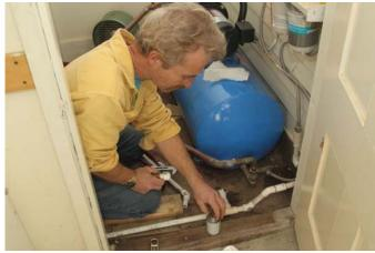
Dave Prowten replacing the broken drain valve. \*
